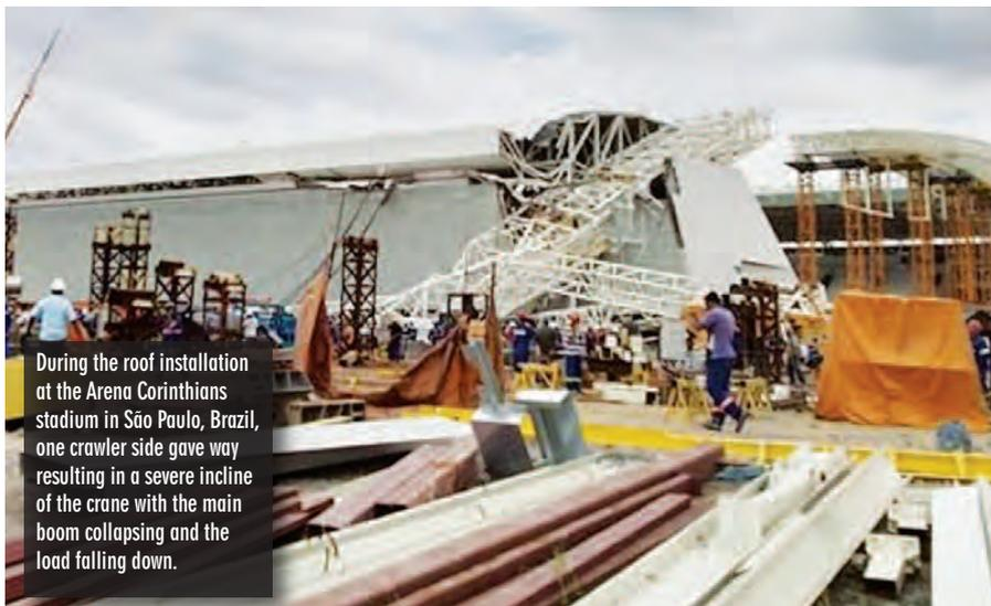
During the roof installation at the Arena Corinthians stadium in São Paulo, Brazil, one crawler side gave way resulting in a severe incline of the crane with the main boom collapsing and the load falling down.
